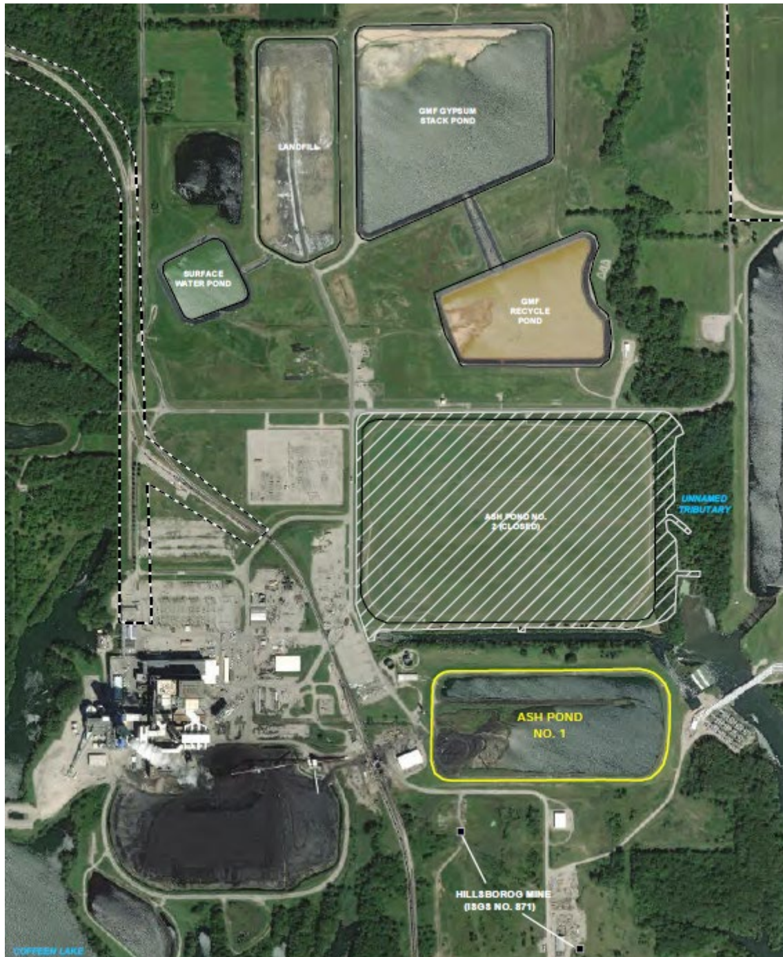
Figure 1.1 Site Location Map. GMF = Gypsum Management Facility. Adapted from Ramboll (2021a).
