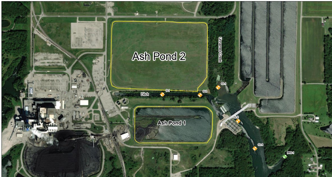
Figure 2.3 Surface Water Sampling Locations. Source: Geosyntec (2021).
